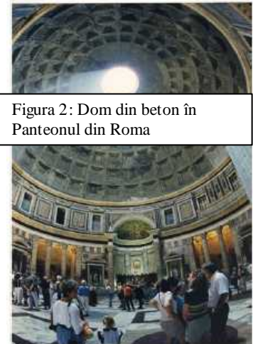
Figure 2: Concrete dome in the Pantheon in Rome
